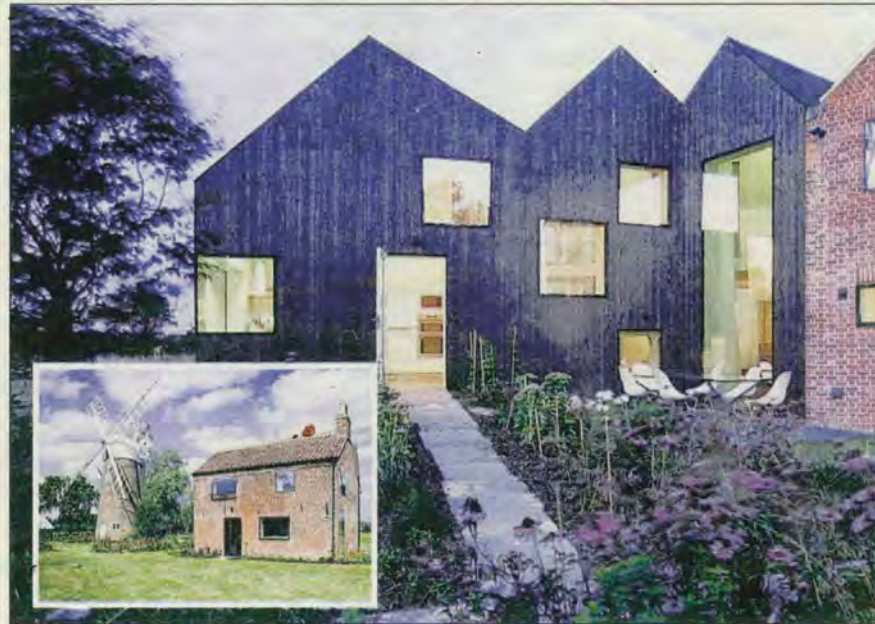
WIND IN THEIR SAILS: The house next to Hunsett Mill, above and inset, which has won an architects' award for the best extension in the country.
